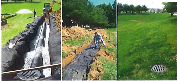
Figure 3: Example of Infiltration Trench Installation
